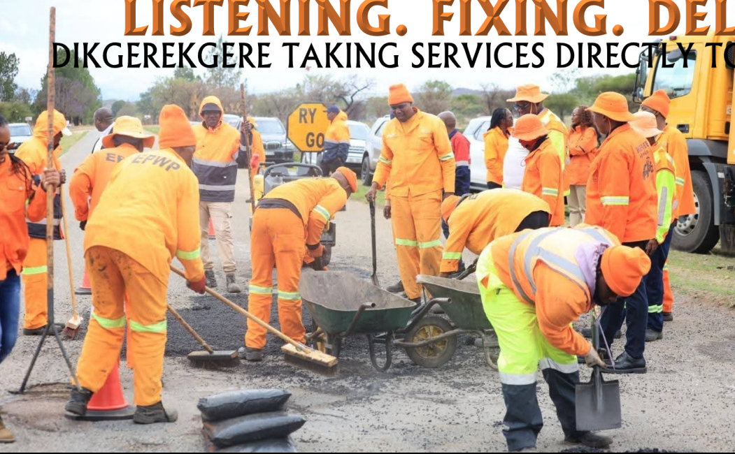
Departmental Pothole Patching team at D2454 Myngenoegen , Dalmada Road
